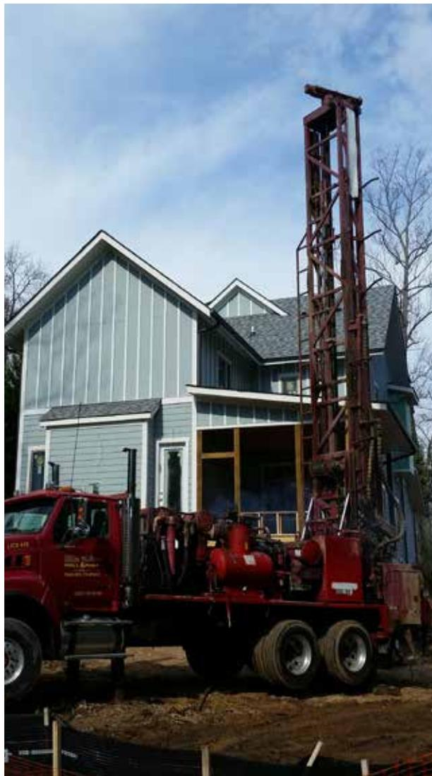
Right: The vertical wells were drilled at the back corner of the home.
