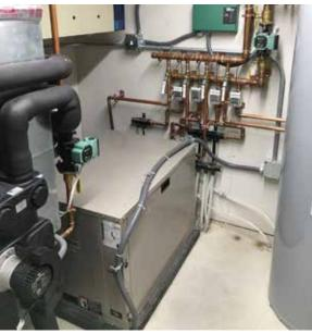
Left: 2-Ton GeoComfort Combination unit Right: 2-Ton GeoComfort Water-to-Water unit
