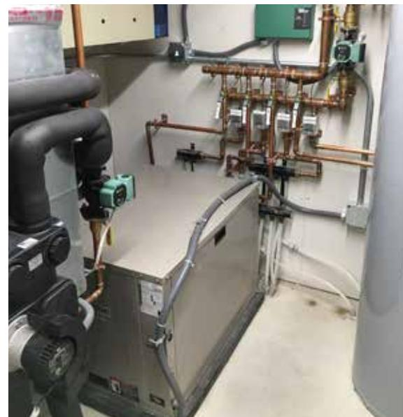
Right: 2-Ton GeoComfort Water-to-Water unit
